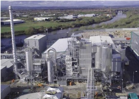
SAICA Partington / UK - 2012 22 MWth heat (20 bar/215°C) rejects, paper fibres, sludge
