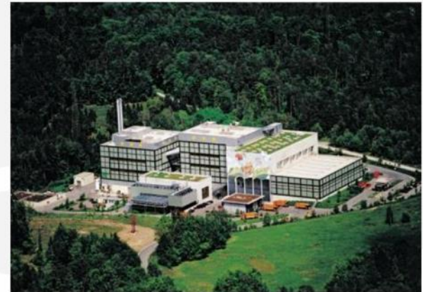
RBB Böblingen / D - 2005 6 MWth (40 bar, 390°C) biomass, wood residues
