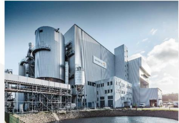
Vattenfall Rostock / D - 2010 87 MWth (42/65 bar, 405°C) grate RDF, municipal- + industrial waste
